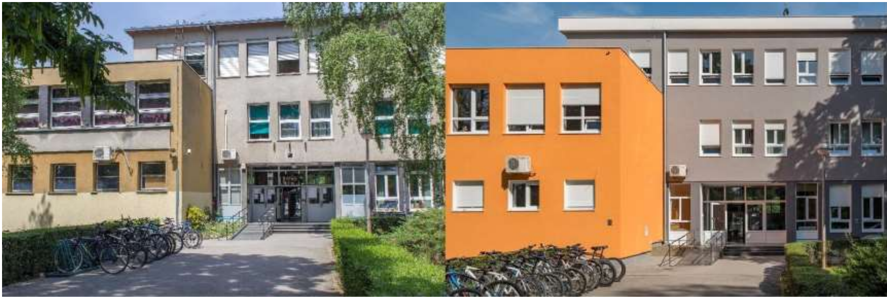
"Ruđer Bošković" Technical School - before and after reconstruction
